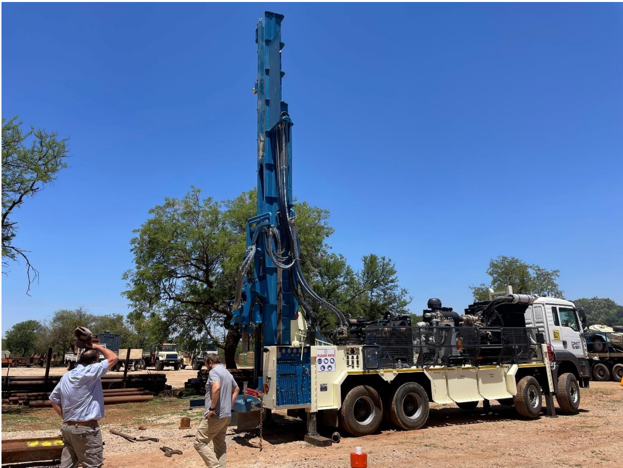
FIGURE 5-1: EXAMPLE OF A DRILL RIG,
