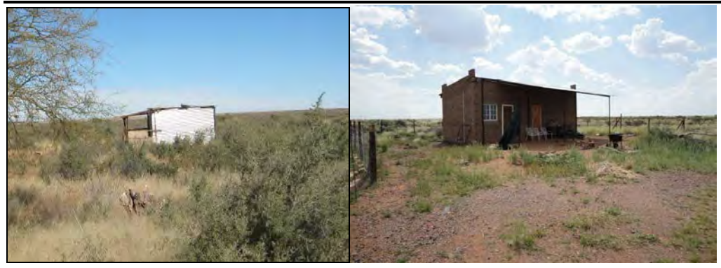
Figure 6.22 Shed built with Corrugated Iron (Left) and Labourers Cottage (Right)
