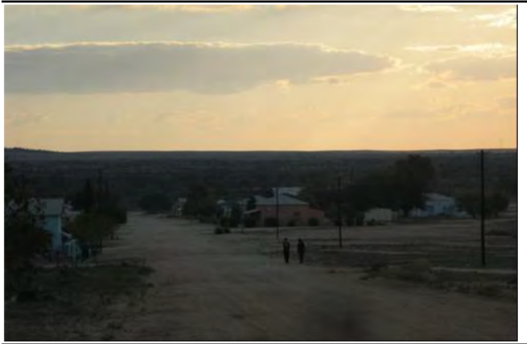
Figure 6.15 Local Secondary Road, Kenhardt
