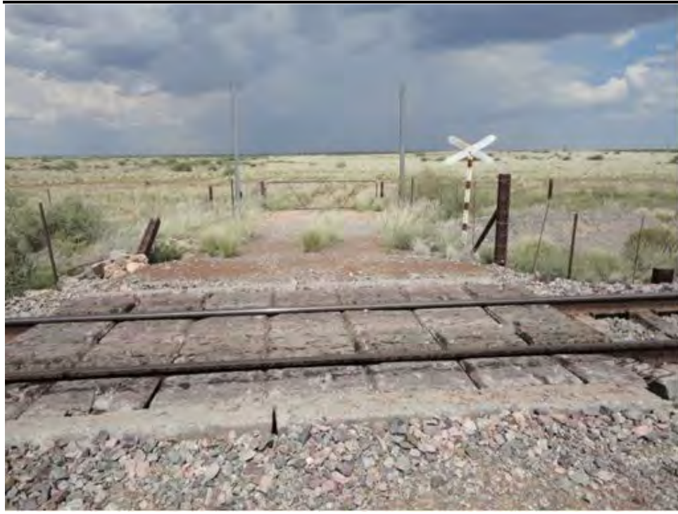
Figure 1.7 Railway Crossing Connecting Two Sections of Olyven Kolk Solar Power Plant Site
