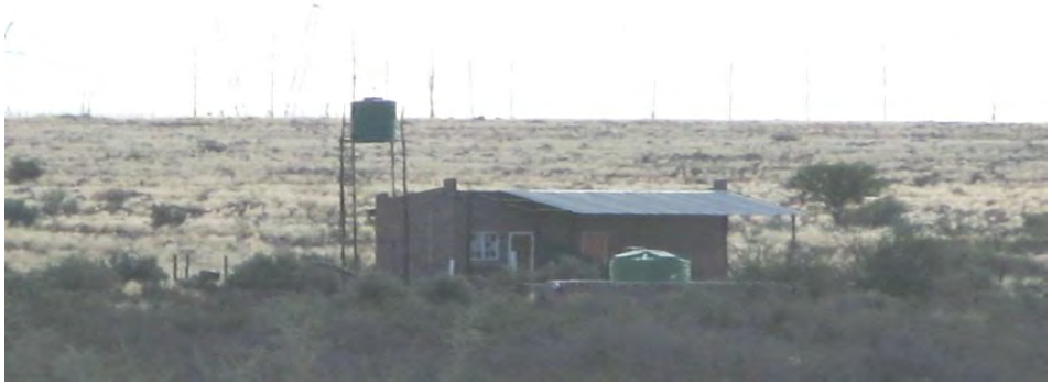
Figure 3: Zoom of existing structure on site (GPS 026)
