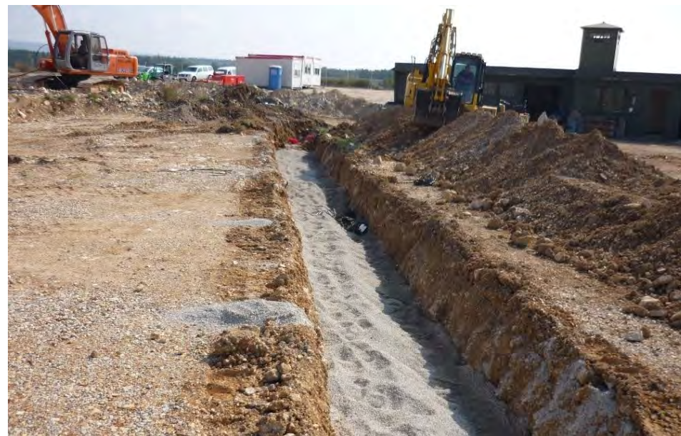
Figure 3: Example trench construction (Source: ERM)
