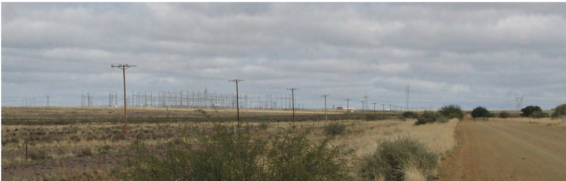
Figure 1: Gravel road sense of place at location with the Aries Substation dominating the landscape context.
