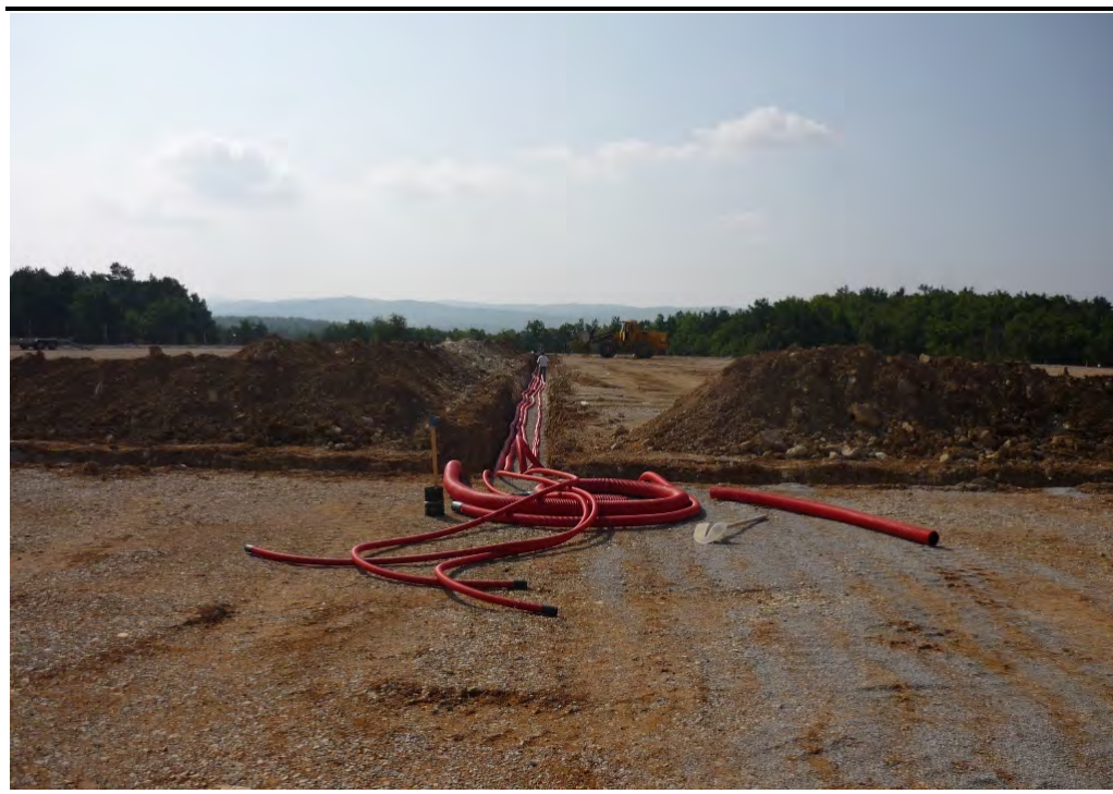
Figure 1.1 Example of Trenching
