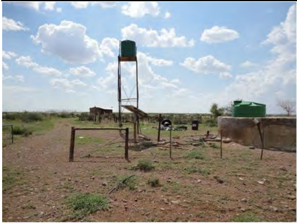
Figure 1.12 View of Existing Borehole on Site
