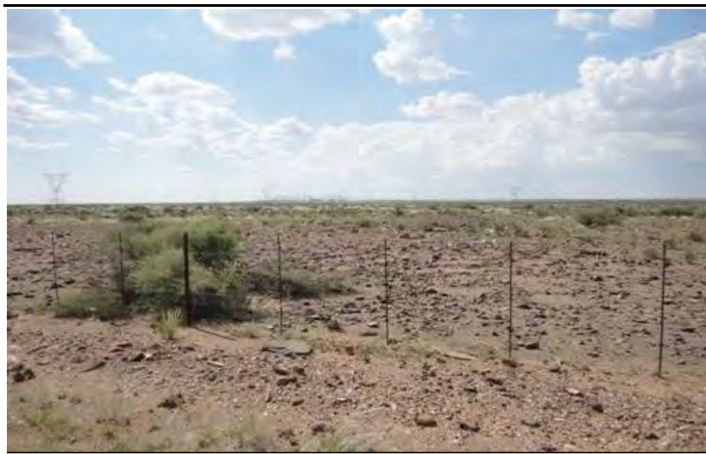
Figure 6.12 Eskom's Aries Substation in the Distance
