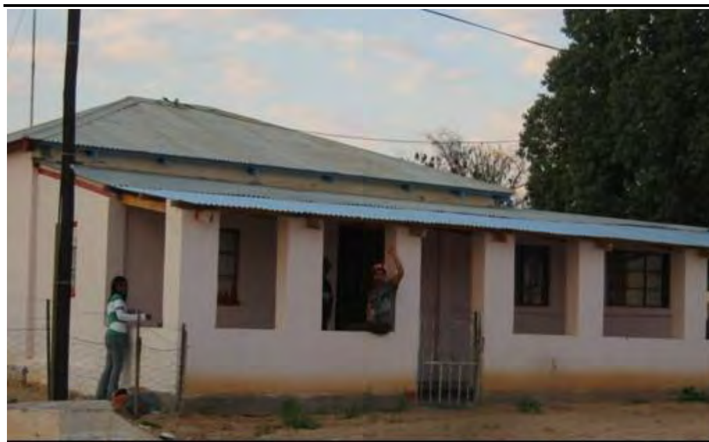
Figure 6.14 House in Kenhardt
