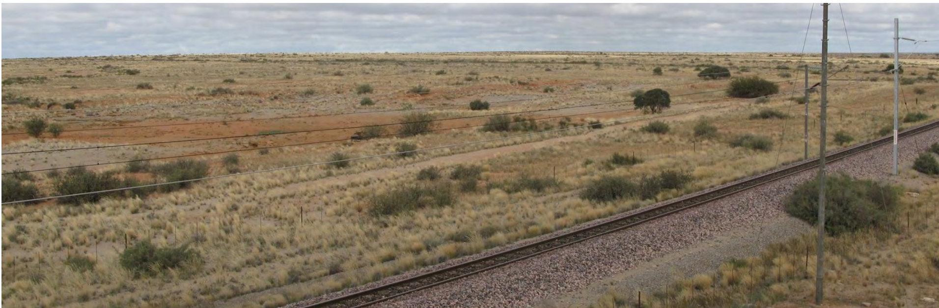
Figure 1: View of existing railway line (GPS 009)
