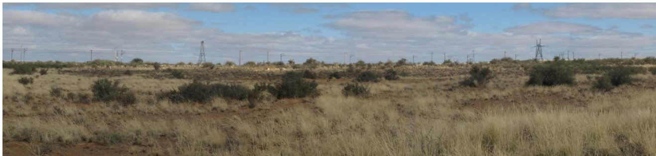
Panoramic view south to south east showing existing vertical nature of the power line modifications to the landscape (GPS 024, Plate 25:GPS Point Map)
