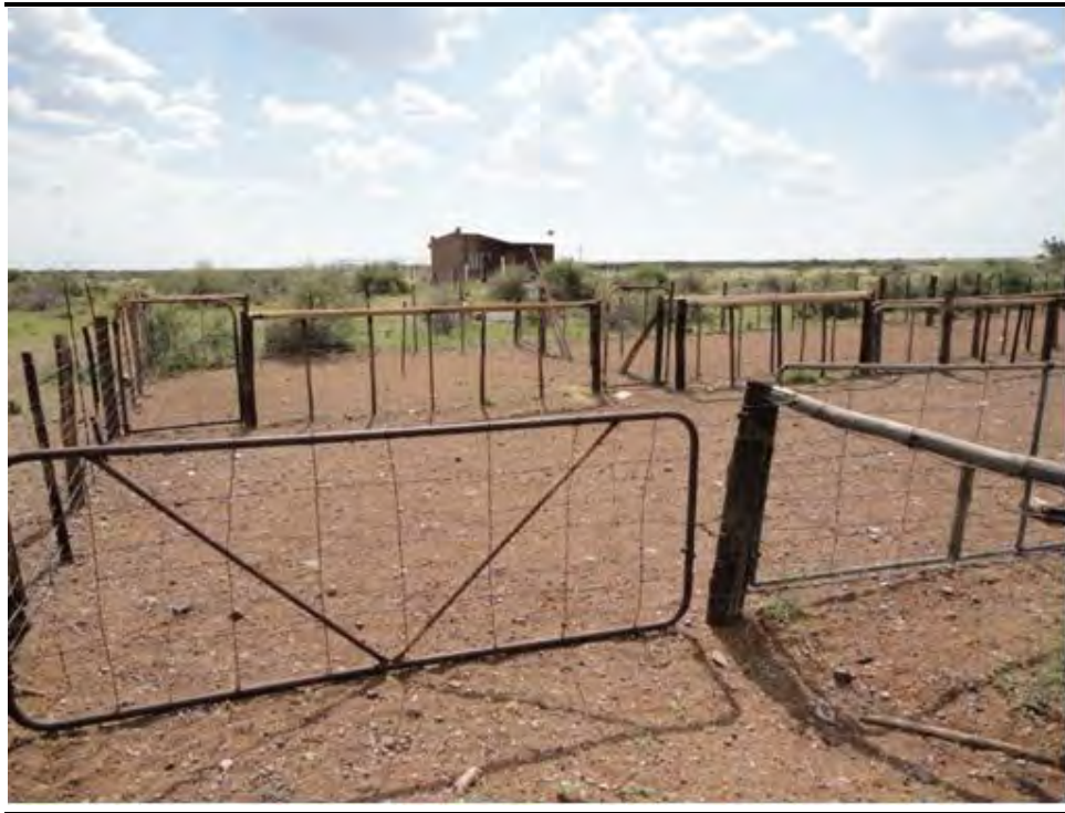
Figure 1.13 View of Derelict Labourers Cottage and Animal Pens
