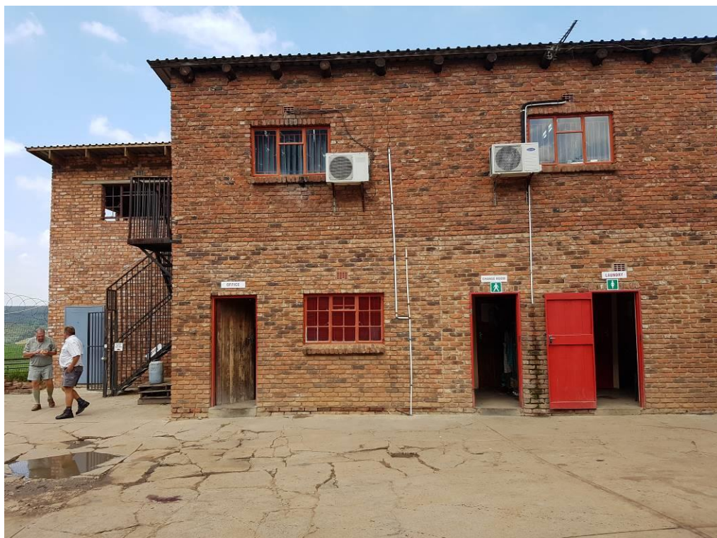
Photograph 1: Example of existing infrastructure including offices, kitchens and ablutions.
