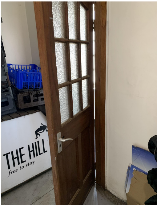
Figure 5.1 Toilet, Internal West Elevation
