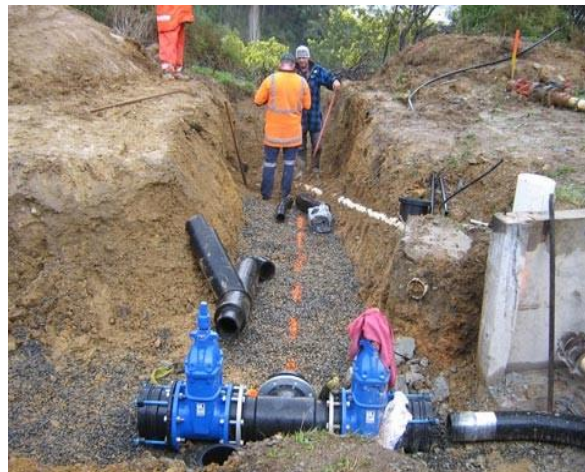
Figure 1: Example of a scour valve
