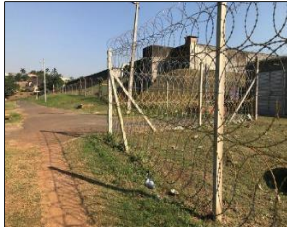
West-facing view, showing the reservoir boundary on the left of the image. The pipeline runs beneath the roads depicted here.
