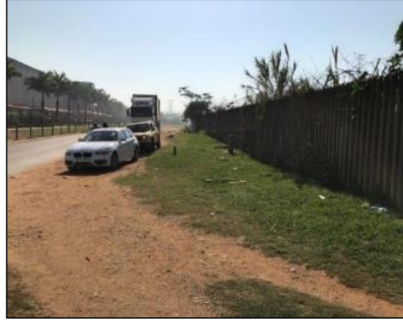
East-facing view , showing the Shoprite warehouse in the top right corner of the image. The new pipeline will be laid on this side of the road.
