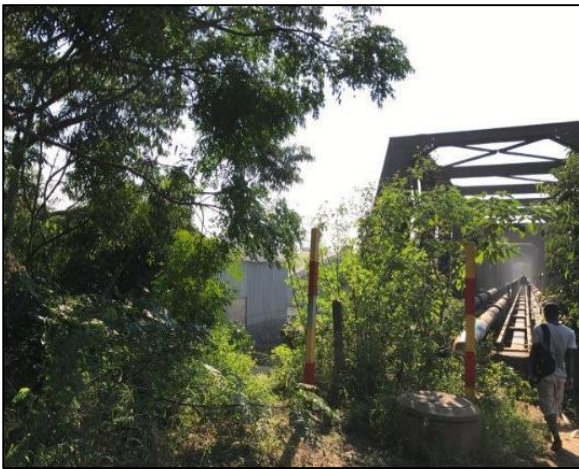
This image depicts the existing pipe bridge with water and 2 sewage pipelines running across. Some of the locals use the bridge as a pass- as depicted here.
