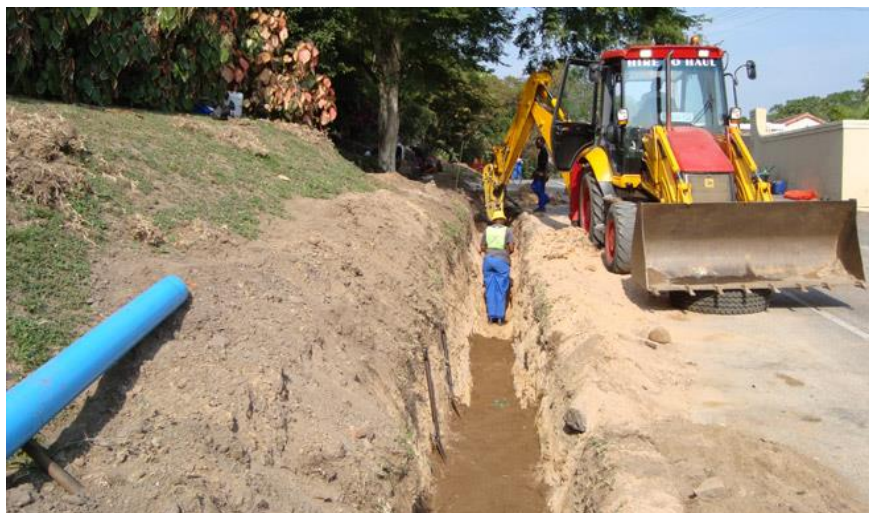
Figure 6: A depiction of a pipeline underlain by riversand bedding
