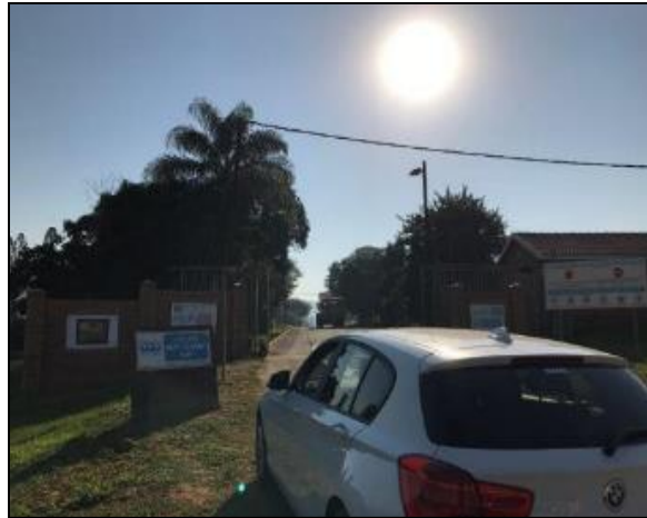
East-facing view, showing the entrance to the WTW.
