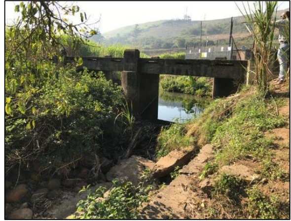
In the conceptual phases, the EWS had considered attaching the new pipeline to the bridge depicted here. However, the structural integrity of bridge has been compromised over the years and the infrastructure damage is noted in a few areas. Hence this option was not favoured. The EWS is proposing the use of pipe jacking at this point.
