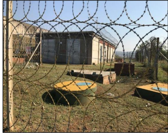
North-west view, showing the reservoir infrastructure.
