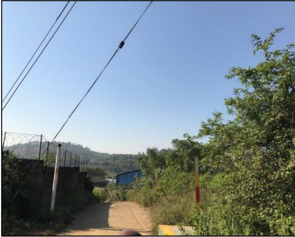
This is one of the points where EWS and Sasol pipeline cross path.
