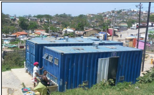
Figure 1: An example of the prefabricated toilets to be constructed within the New City Informal Settlement.
