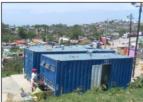
Figure 1: An example of the prefabricated toilets to be constructed within the uMlazi E Informal Settlement.
