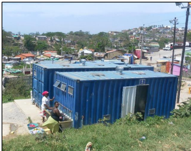
Figure 1: An example of the prefabricated toilets to be constructed within the uMlazi E and V settlement.
