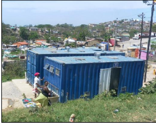
Figure 1: An example of the prefabricated toilets to be constructed within the uMlazi E and V settlement.
