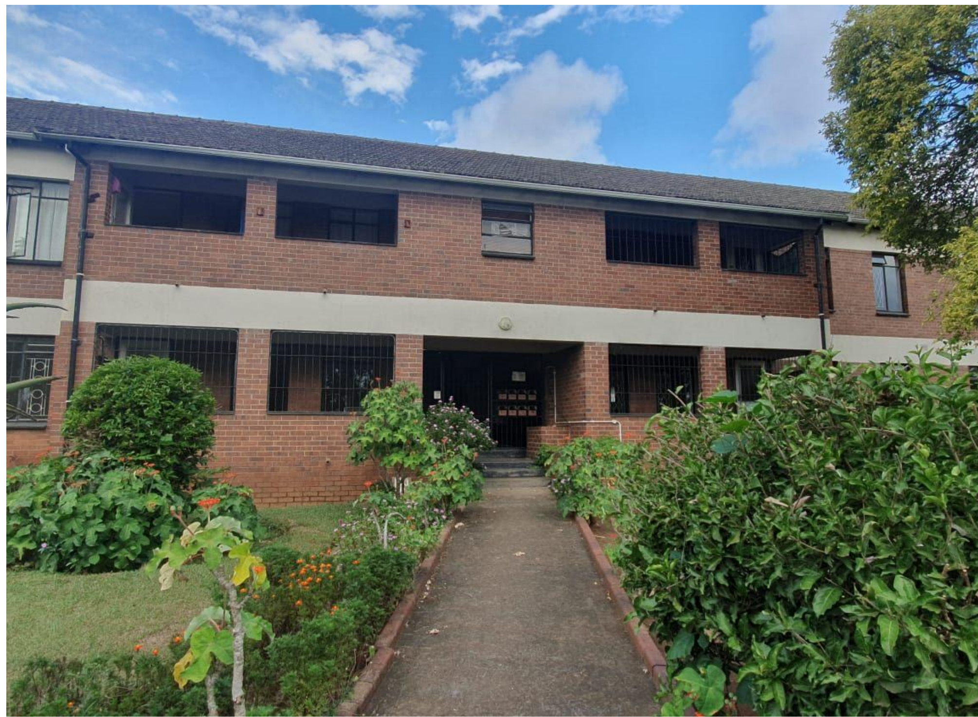
EXISTING BLOCK - CHRISTIE RD VIEW
