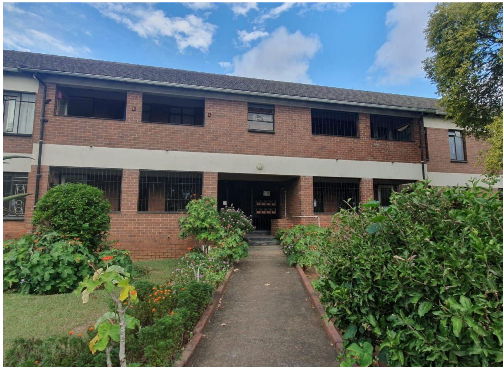
EXISTING BLOCK - CHRISTIE RD VIEW
