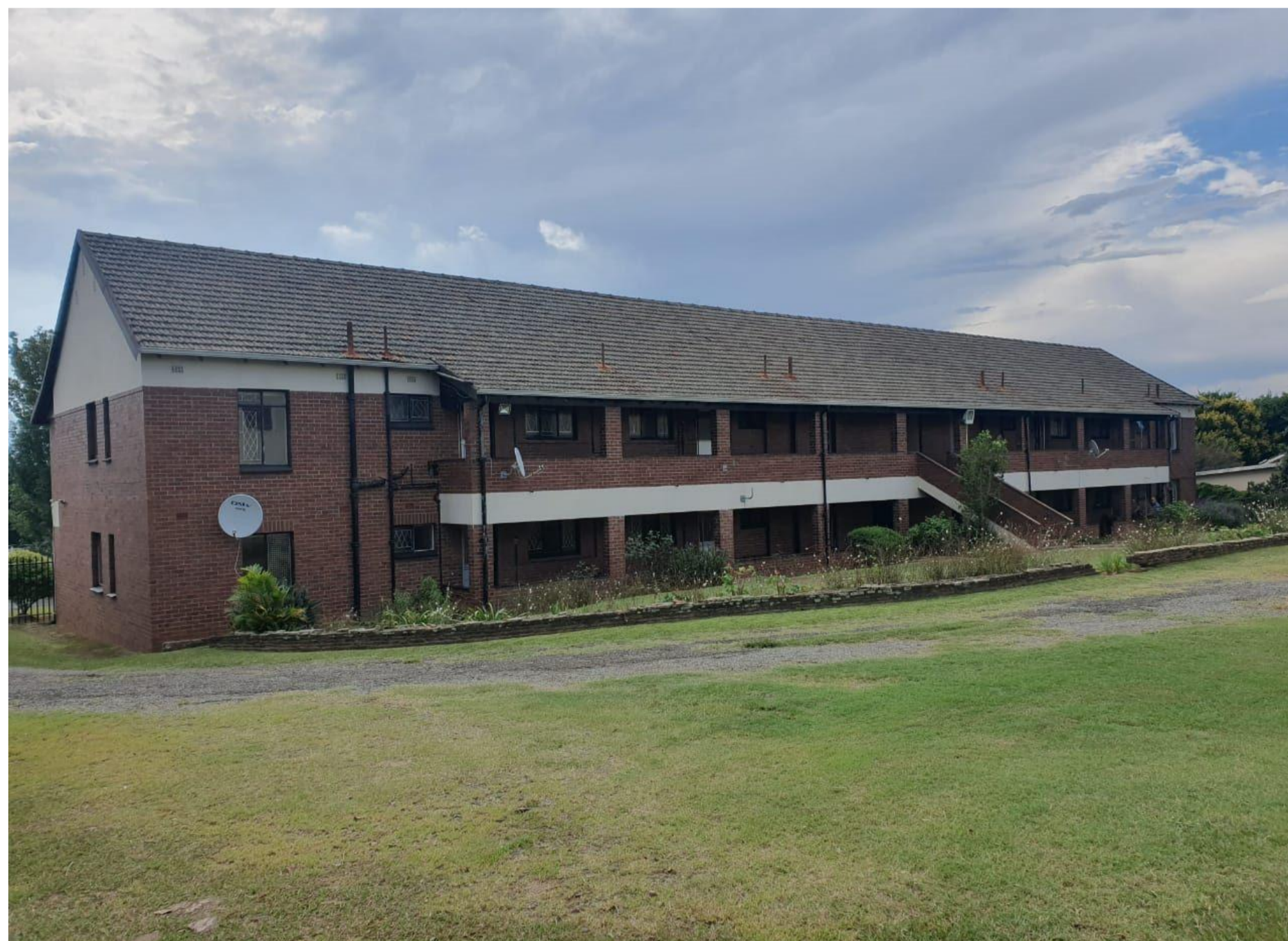
EXISTING BLOCK - CHRISTIE RD VIEW
