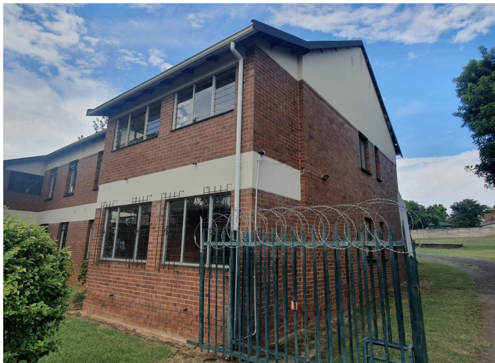
EXISTING BLOCK - CHRISTIE RD VIEW
