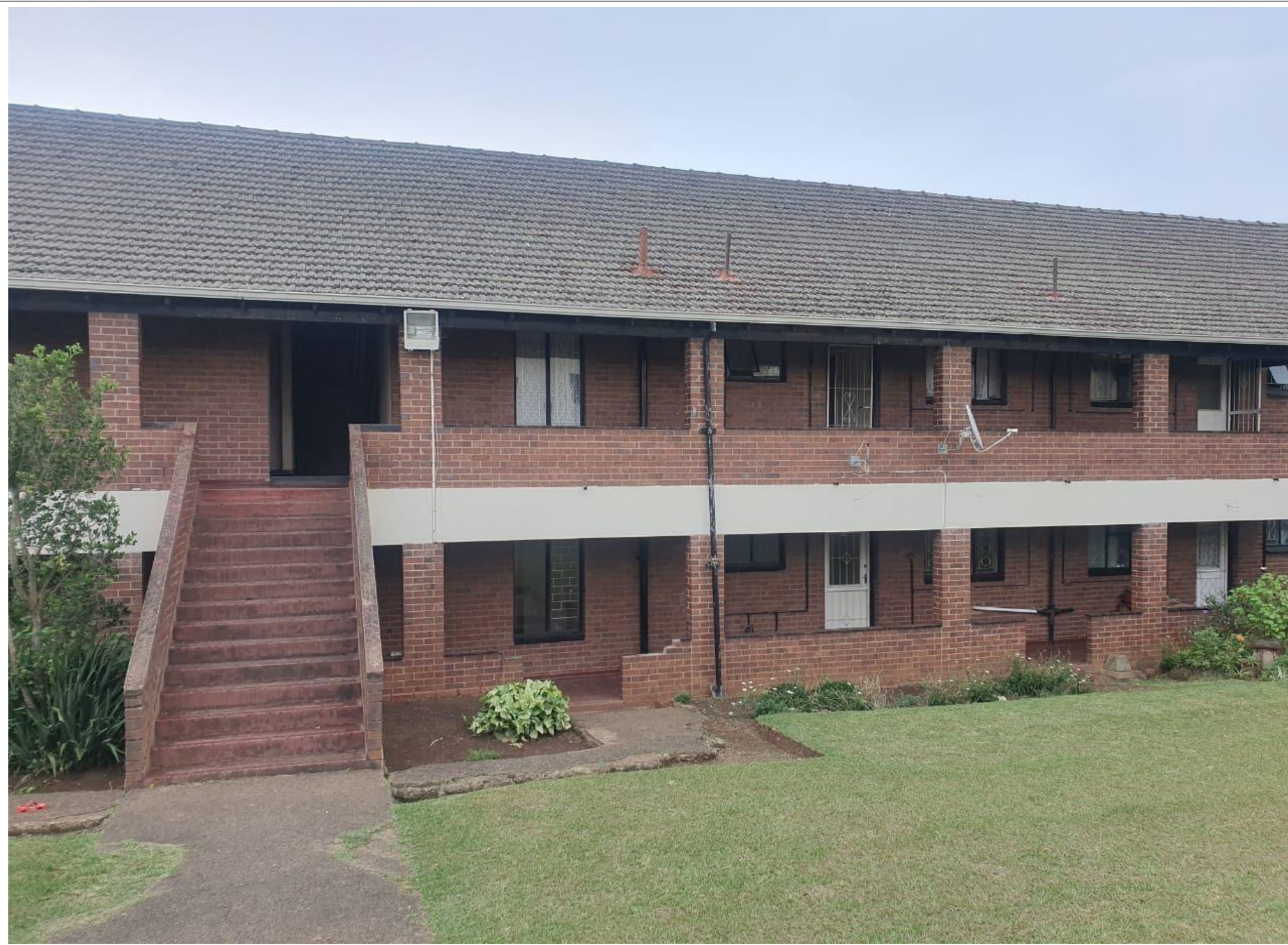
EXISTING BLOCK - CHRISTIE RD VIEW
