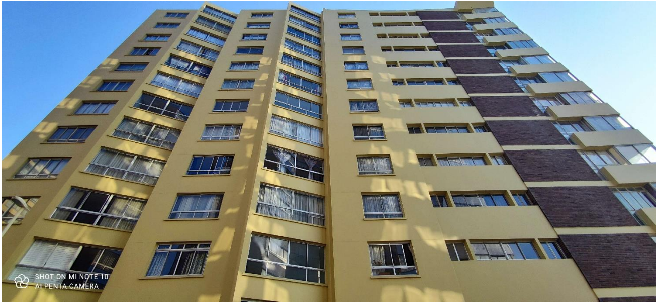
Figure 5. Image illustrating the side façade perspective upwards (East Elevation). No work to be undertaken externally.
