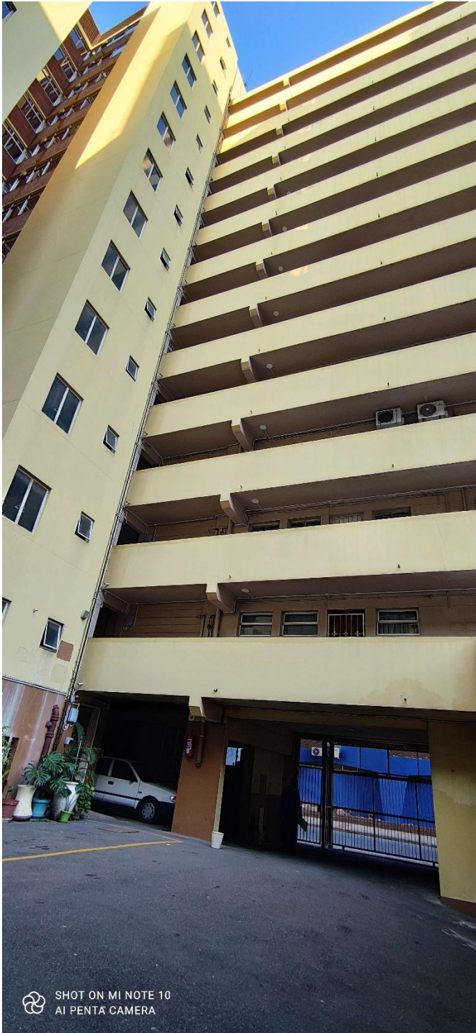
Figure 8. Image illustrating the side façade (north West Elevation) and part rear faced (South West elevation). No work to be undertaken externally.
