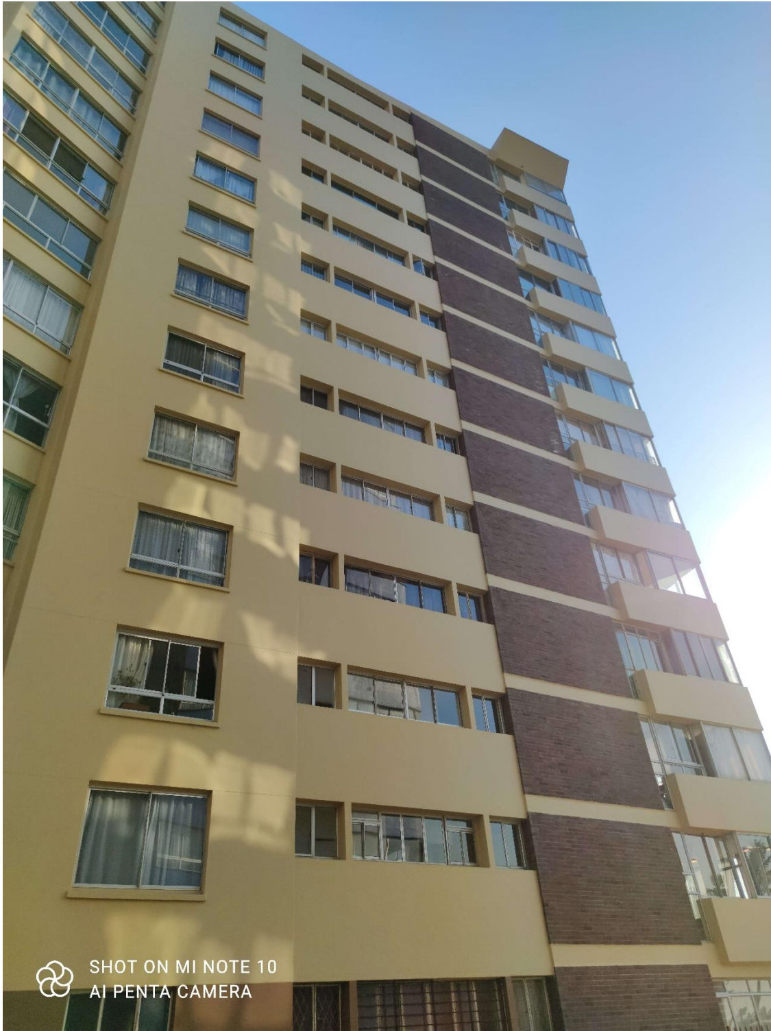
Figure 3. Image illustrating the part side façade (East Elevation). No work to be undertaken externally.
