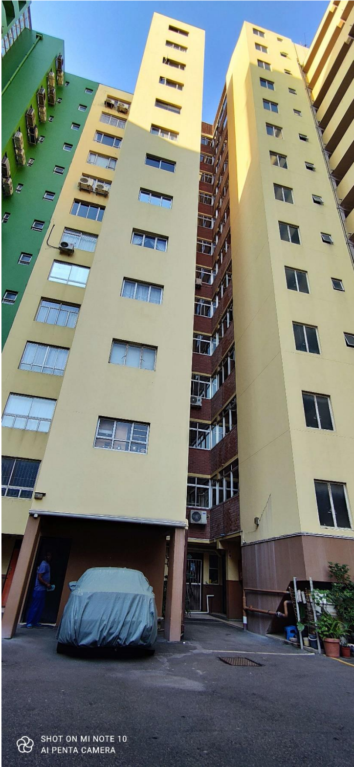
Figure 9. Image illustrating the side façade (South West Elevation). No work to be undertaken externally.
