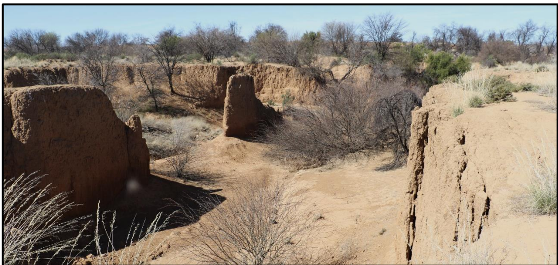
Figure 7. Very deep erosional features occur along the drainage network on the alluvium.
