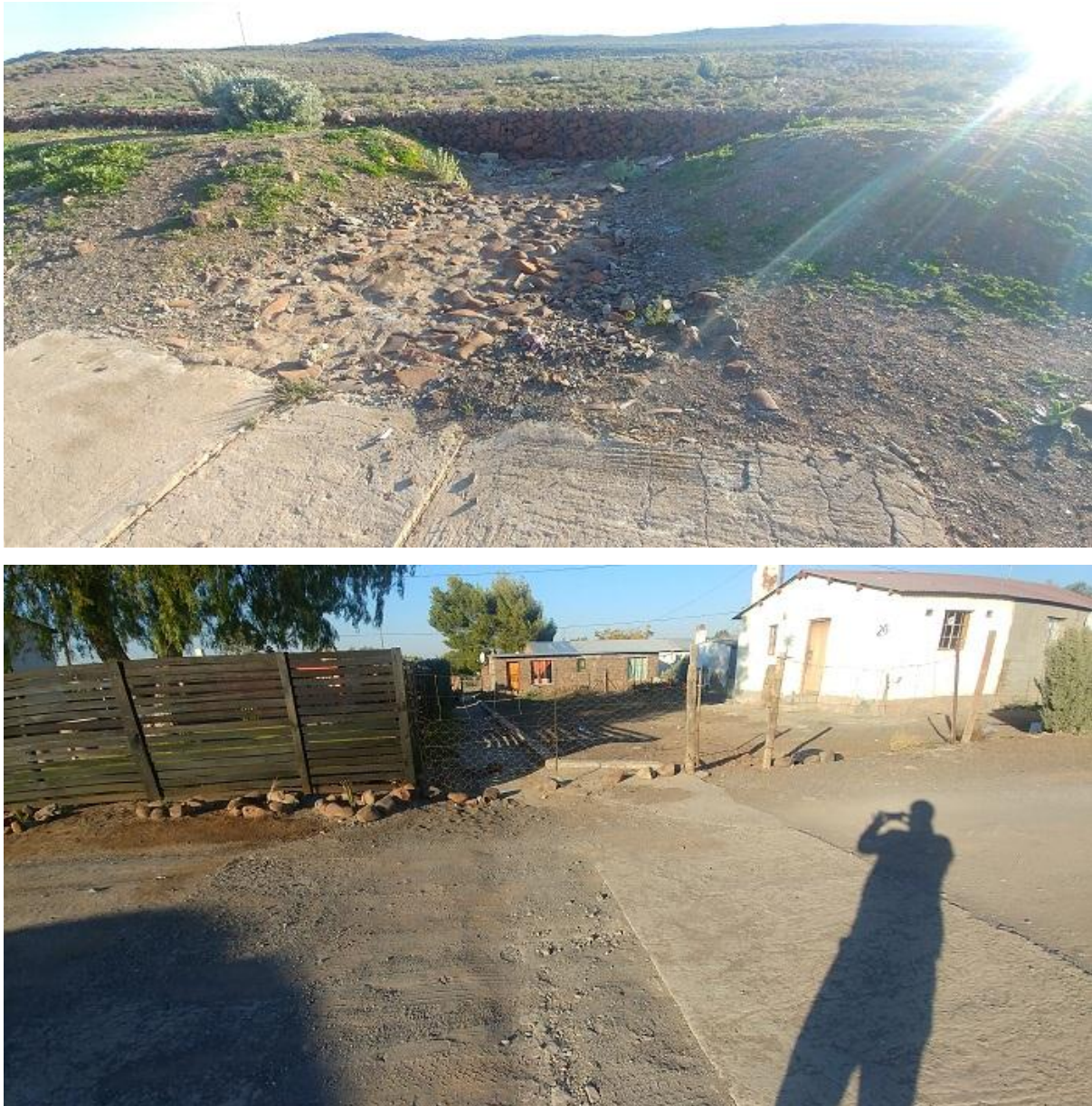
Figure 9: Two images illustrating the artificially constructed surface water drainage channels which drain surface water runoff through the informal settlement towards the south
