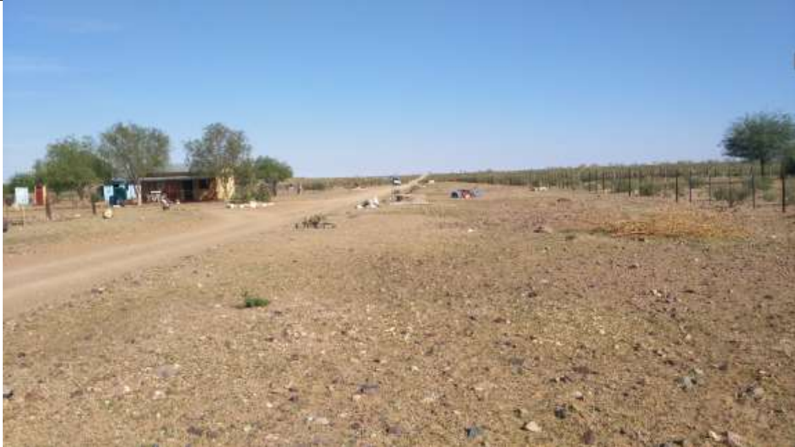
Figure 9 View of pipeline footprint, in Swartkopdam (km 0 of survey transect)
