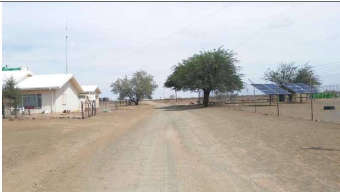
Figure 22 Noenieput, where the pipeline starts (end of survey)
