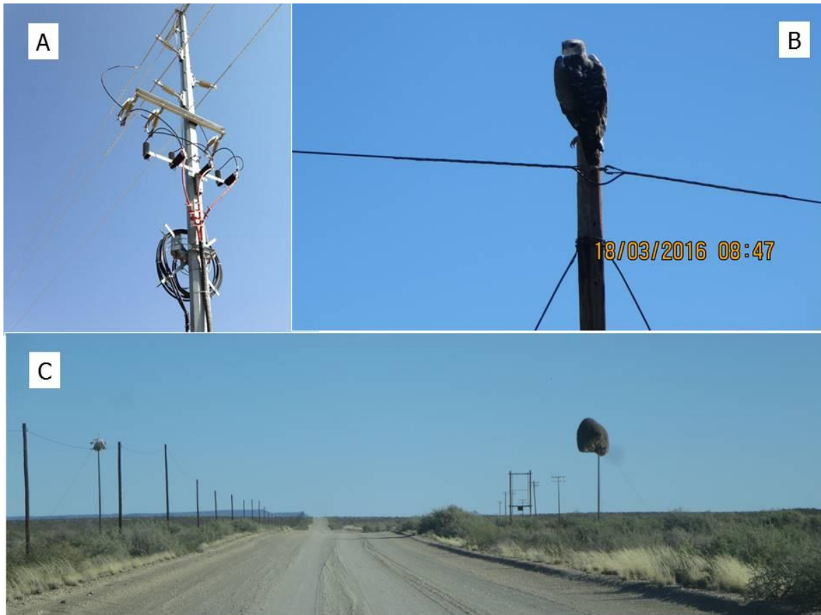
Figure 18: Electrical overhead infrastructure that is attractive to some species of birds as perches or nest sites. (A) insulator carriers and cables that provide nesting sites for birds (photo supplied by CSIR), (B) Martial Eagle perched on a pole near Carnarvon, (C) Sociable Weaver nests on electrical infrastructure near the SKA Core area on the Carnarvon-Van Wyksvlei road (Photo SJ Milton)
