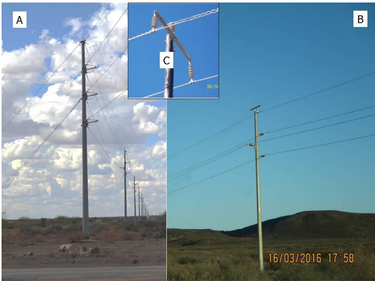
Figure 16: Designs of overhead infrastructure carrying optic fibre and cables (A & B) steel monopoles, (C) wood monopoles (Photos by Lydia Cape)
