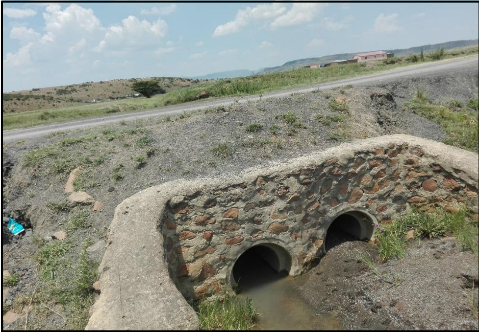
Figure 2 Showing: Existing Pipe Culverts
