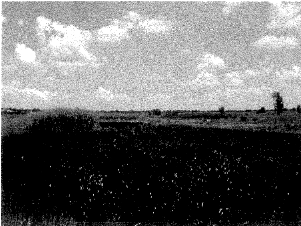
Figure A16: Upstream view from N4 highway of culverts along a tributary of the Brugspruit at River Crossing 6
