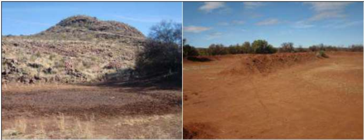
Figure 10: The dams BP01 and BP02 both of these are constructed sand dams that hold water when water flows
