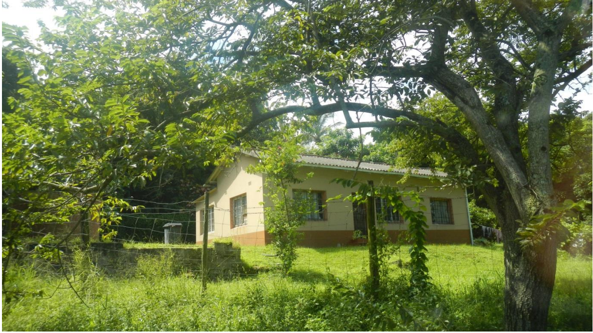
Figure 8: Outside view of the heritage building outside of the proposed project area
