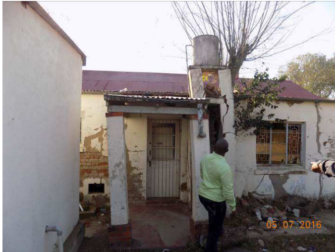
Figure 12: South Western Facade with tree growth in wall
