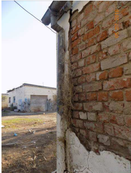
Figure 10: Shows the cracks and exposed brickwork
