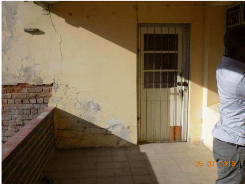
Figure 8: Veranda space showing plaster cracks
