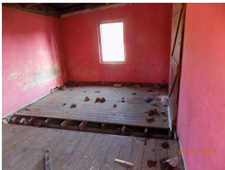
Figure 23: shows the interior of the outbuilding
