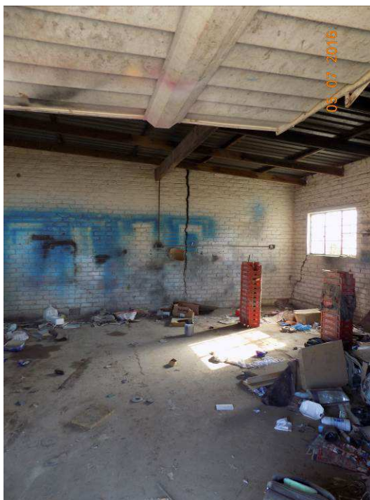
Figure 25: Interior of garage showing large crack
