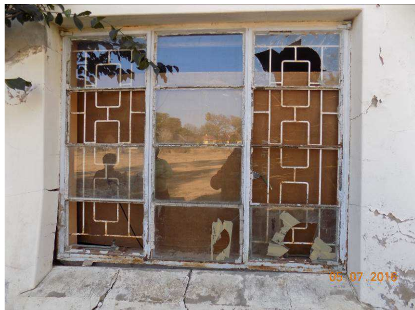
Figure 9: Typical painted steel window
