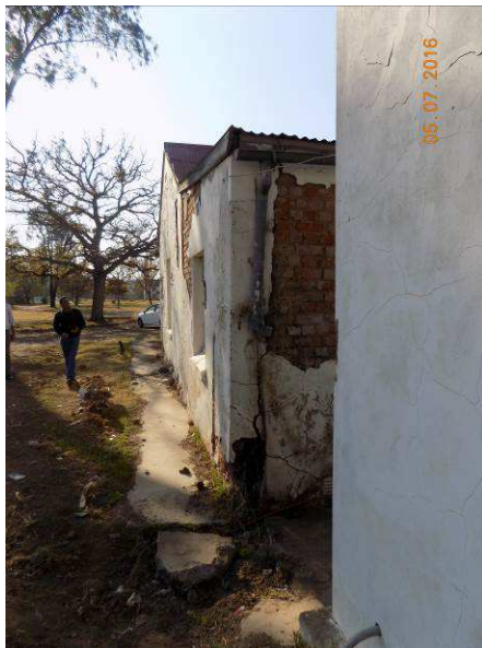
Figure 11: North West corner severely damaged and collapsed
