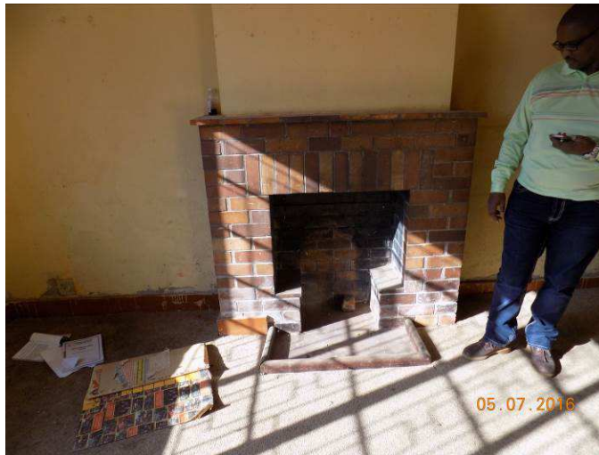
Figure 18: Show existing fireplace
