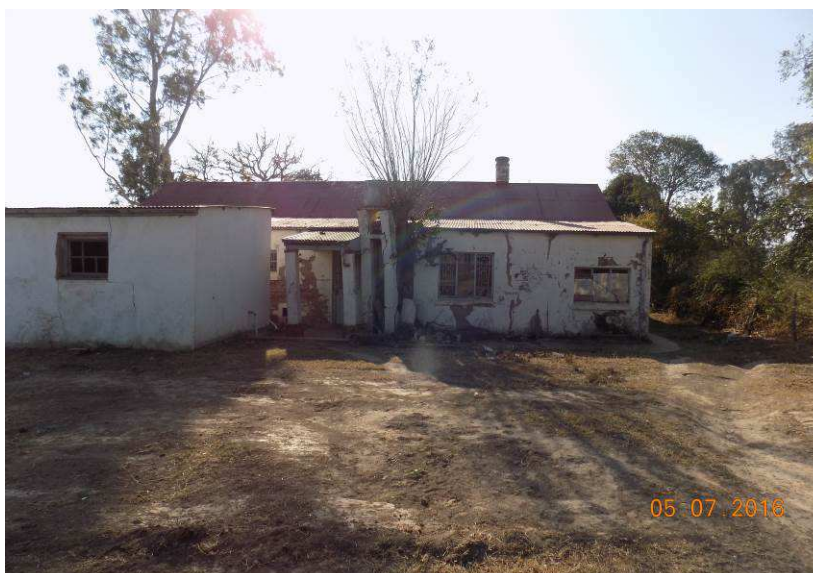
Figure 5: South West facade (back of main house)
