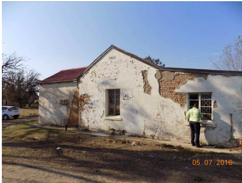
Figure 6: North West Facade with foundations compromised
