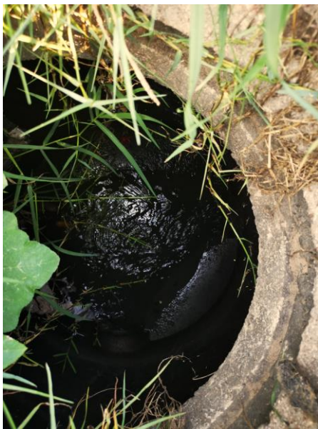
Figure 16 Open sewer manhole on 200mm line
