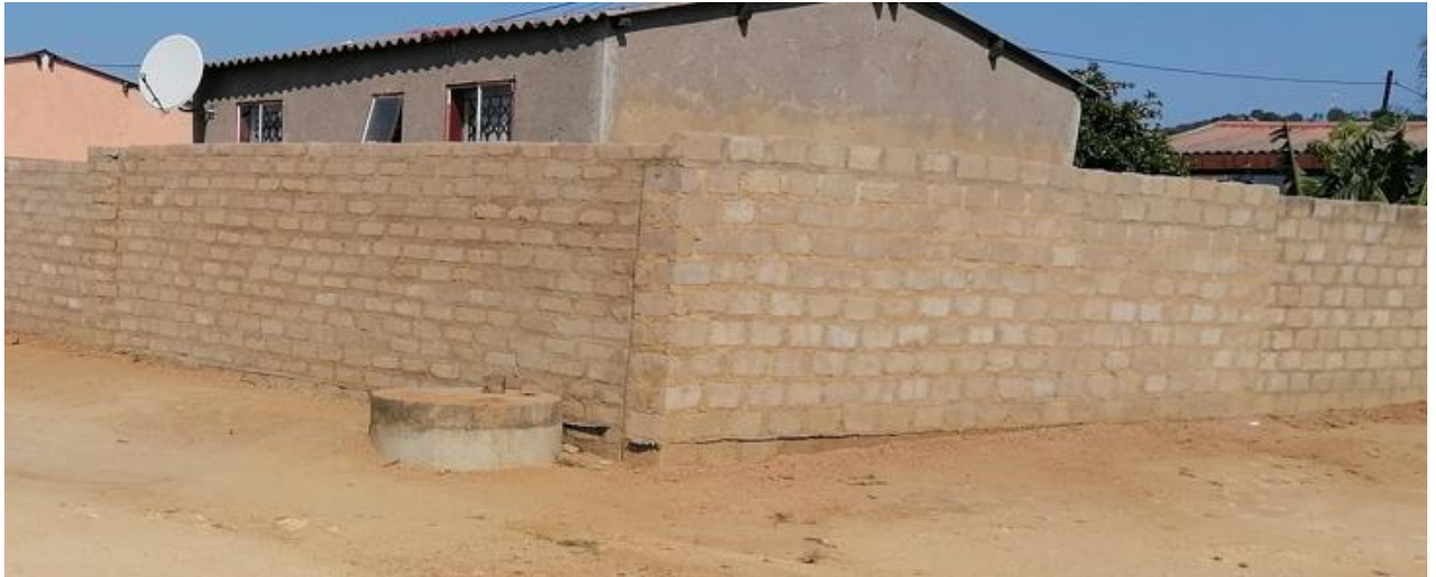
Figure 15 Existing manhole on existing settlement near site
