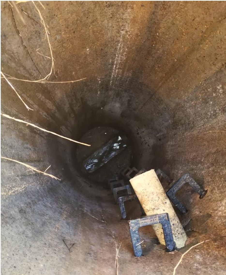
Figure 14 Existing gravity manhole with 300mm diameter sewer outfall
