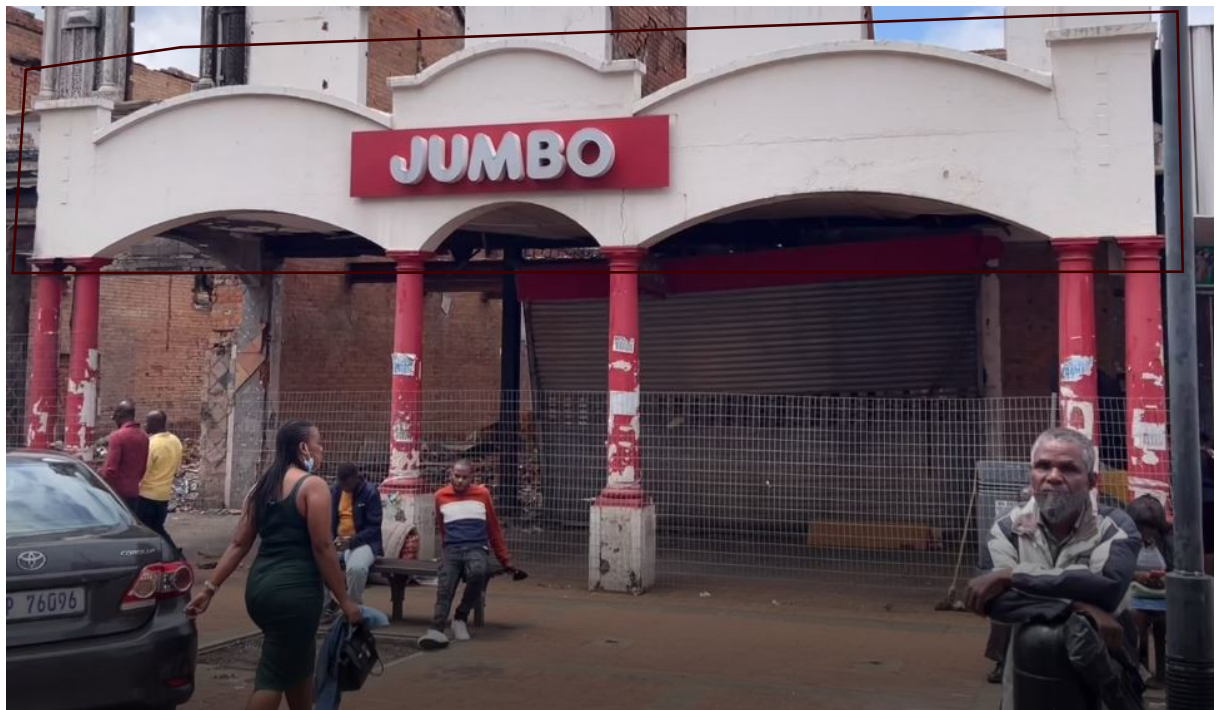
180 Church str facade to be retained
