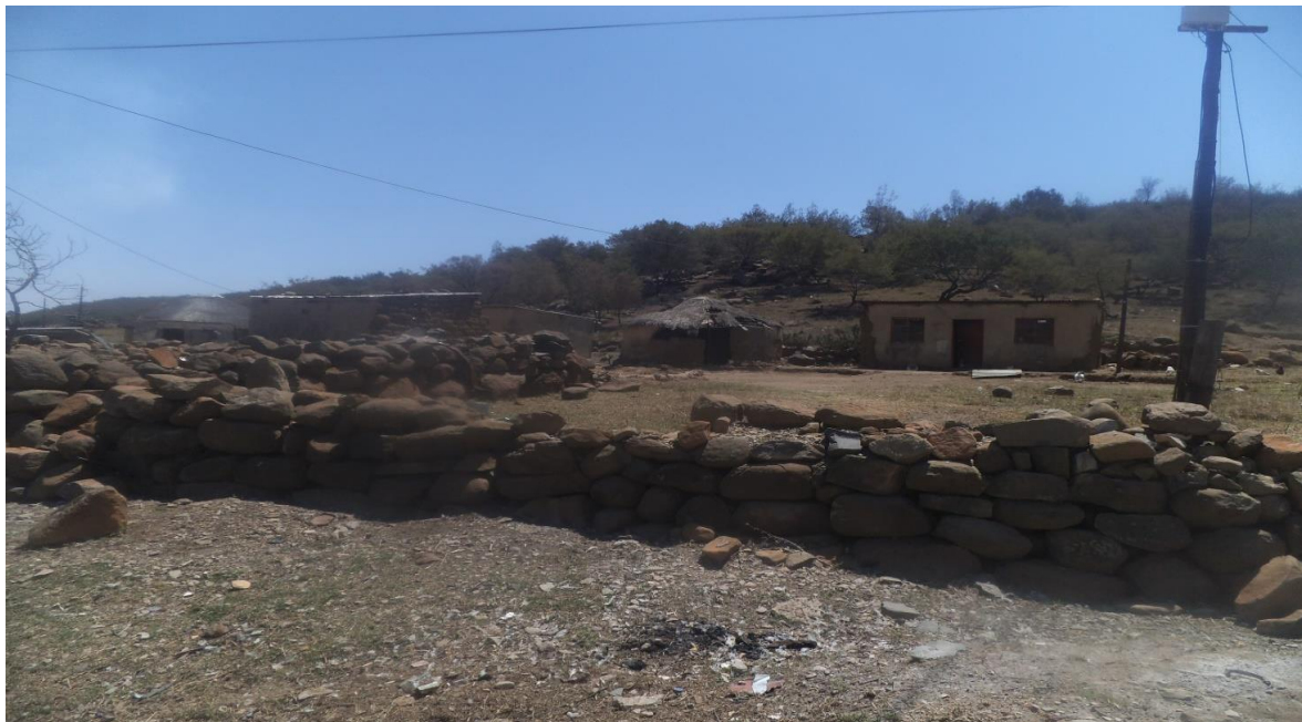
FIGURE 2: IMAGE SHWOING THE STRUCTURE OF THE EXSING HOUSES IN THE AREA
