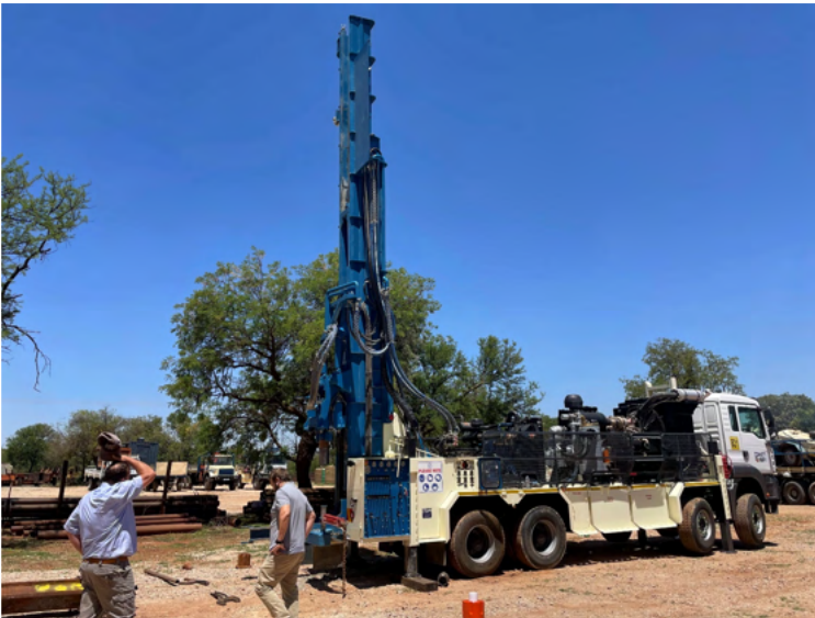
Figure 5-18: Example of a drill rig, (Source: Torque Africa)
