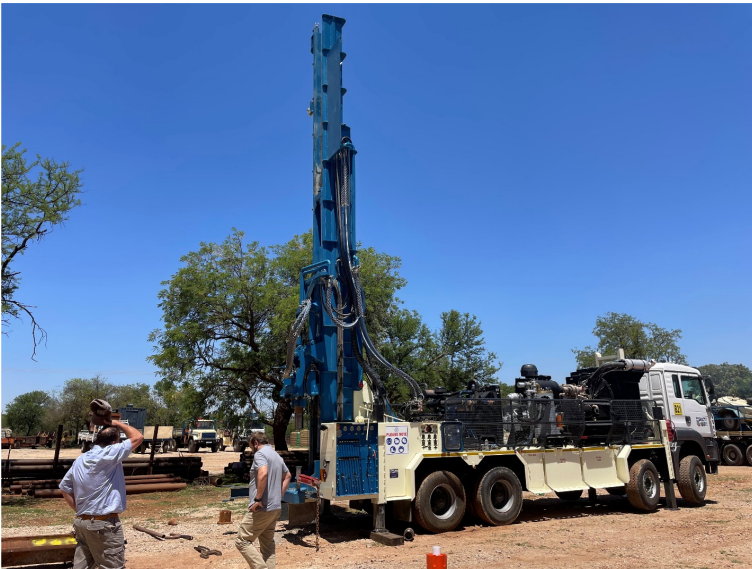
Figure 5-8: Example of a drill rig, (Source: Torque Africa)
