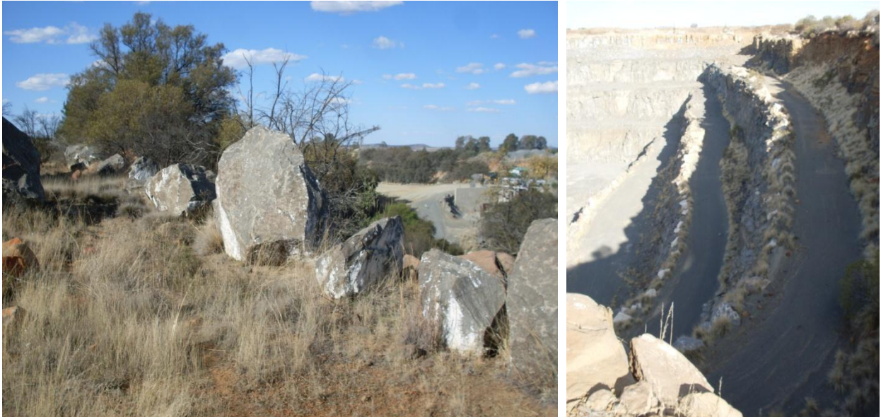
Figure 7 : Placement of big boulders along the crests serve as protection and natural barriers.
