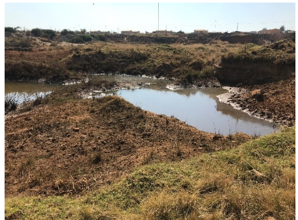
An area to the south of the village where excavations resulting from sand winning and/or historical borrow pits that has resulted in transformation of wetland zones.
