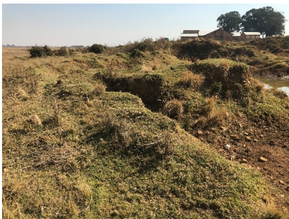
Another view of the excavated area showing the level of landscaping.
