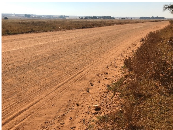
A section of the road to be rehabilitated.
