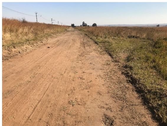
An existing gravel road that runs parallel to the existing railway, which is used largely as a service road as well as an access for the agricultural sector.
