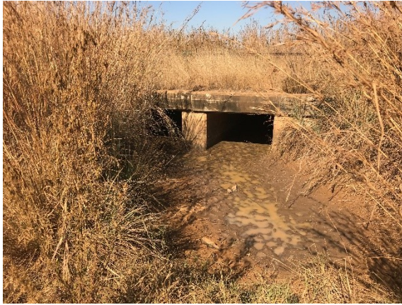
Existing bridge/culverts. This allows surface water drainage beneath the existing railway.
