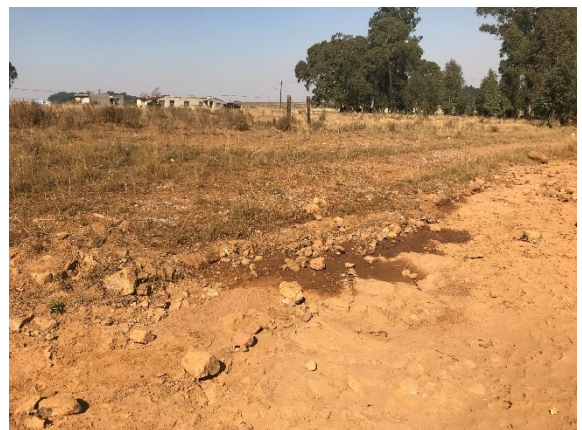
A section of the road that was constructed within wetland habitat that has completely altered the functionality of the wetland area. Wetland seepage still occurs within some areas to drain within the road reserve.
