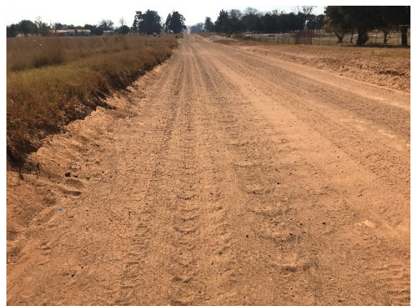
Another section of the roadway that is to be rehabilitated.
