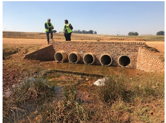
The bridge design of the main watercourse, showing the series of side-by-side culvert pipes.
