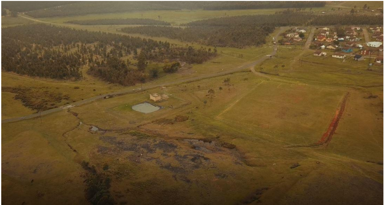
Photo 2.3: Existing pump station and sports field within the project area
