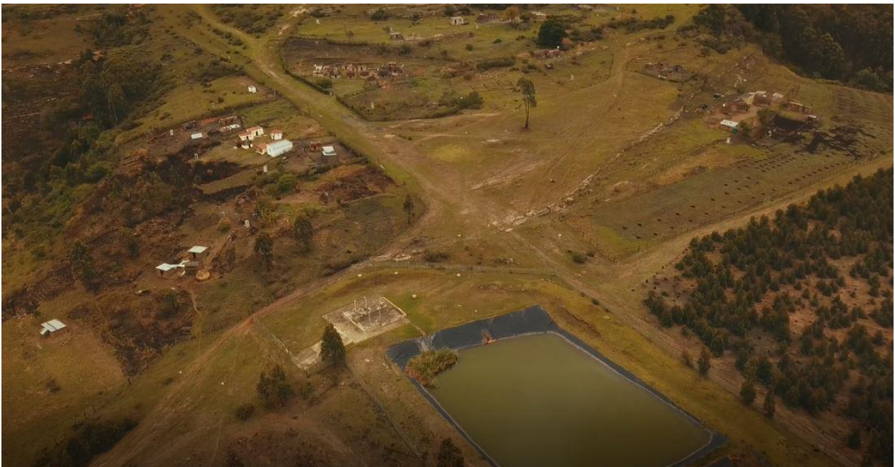
Photo 2.2: Existing traditional dwellings, vacant pockets of land and wastewater treatment plan
