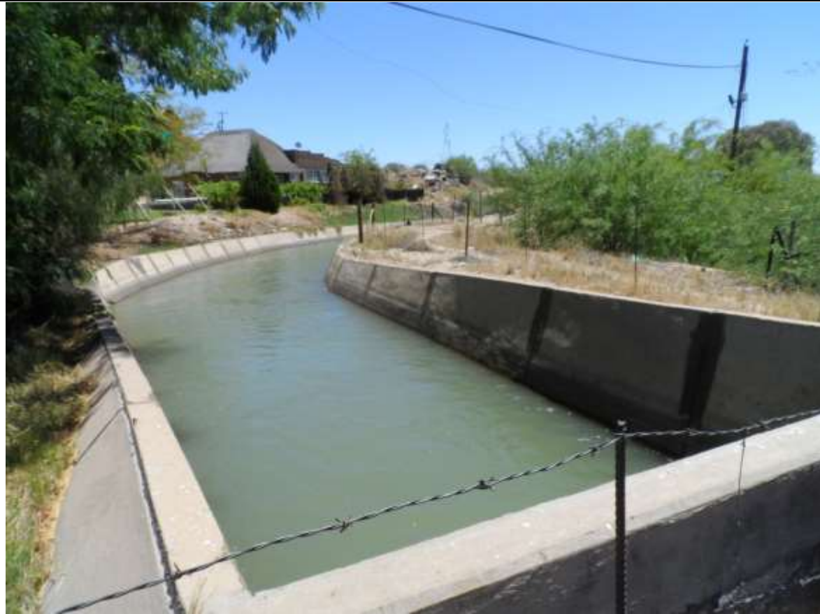
Figure 3: View of the canal crossing the property, looking west.
