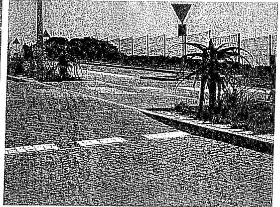
Raised pedestrian table along the Triple Point Access Road
