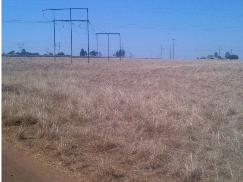
Photo 3 :The new Line 2 will be constructed on the right hand side of this line that would be dismantled – photo taken in a southerly direction
