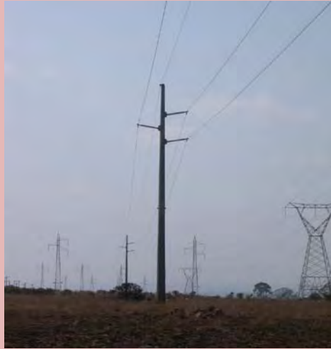
Figure 2: 132 kV steel monopole structure
