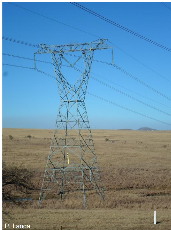
Figure 9: Example of a self-supporting suspension tower (132 kV)
