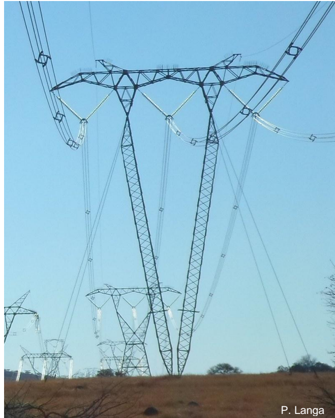
Figure 6: Example of a Guyed-V tower (400 kV)
