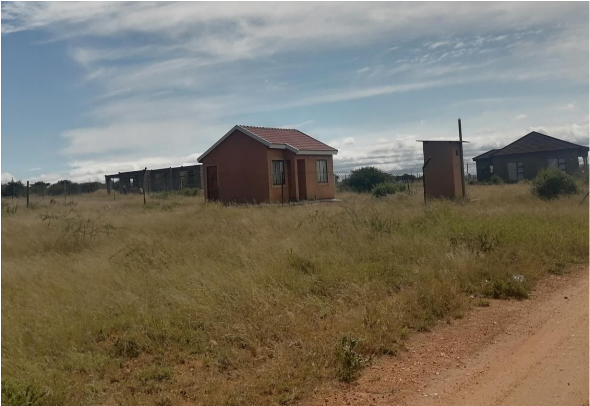
Houses without electricity
