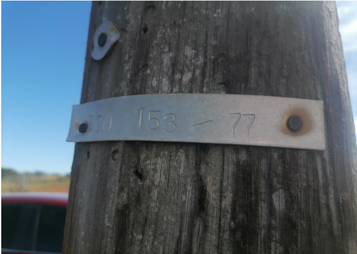
The existing pole number on site
