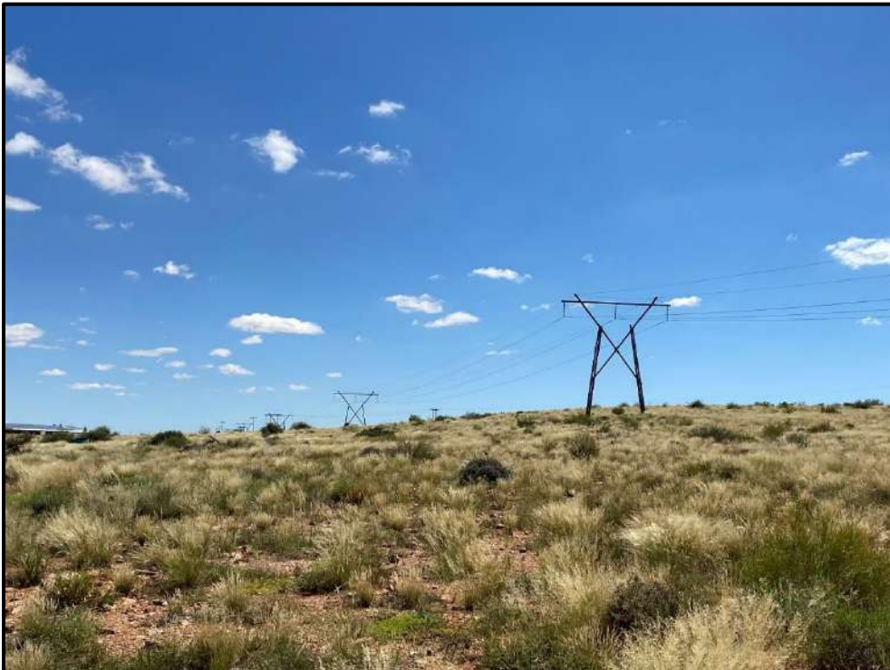
An Eskom powerline traverses the southern section of the project site.
