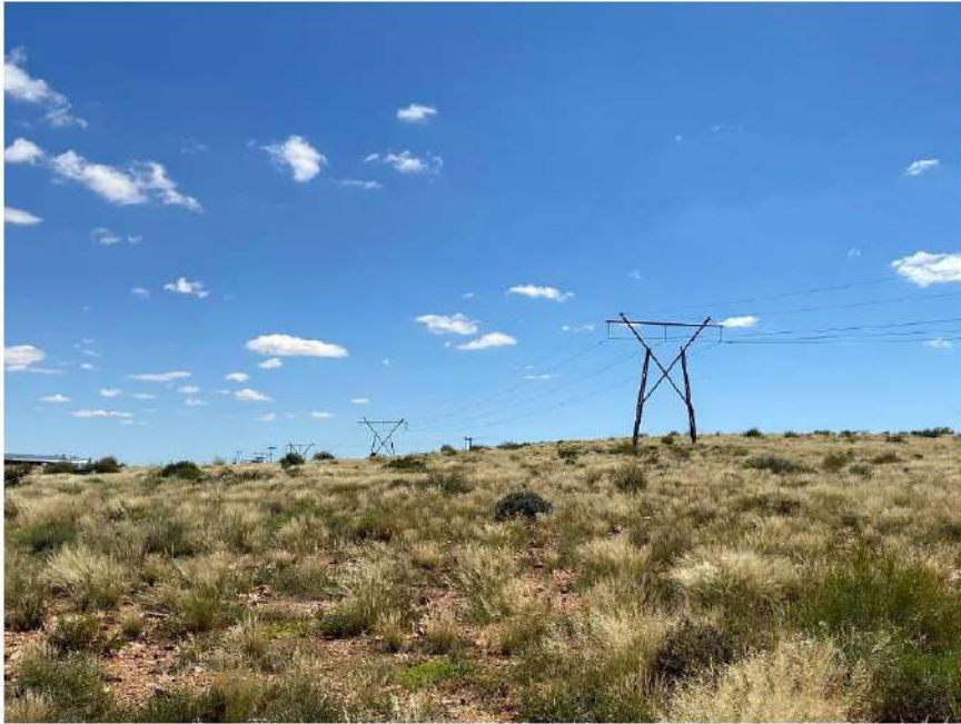
Figure 3.3: An Eskom powerline traverses the southern section of the project site.
