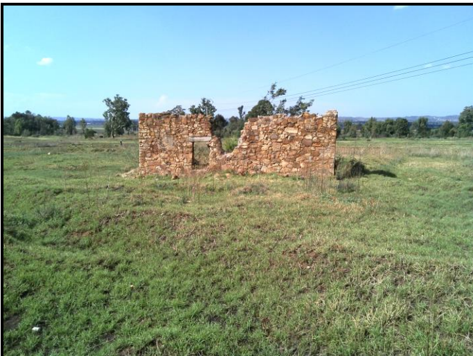
Figure 9: Ruin at Field Number 640 viewed from the south.
