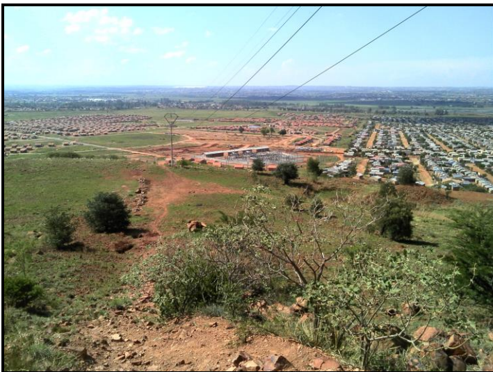
Figure 5. General site conditions.
