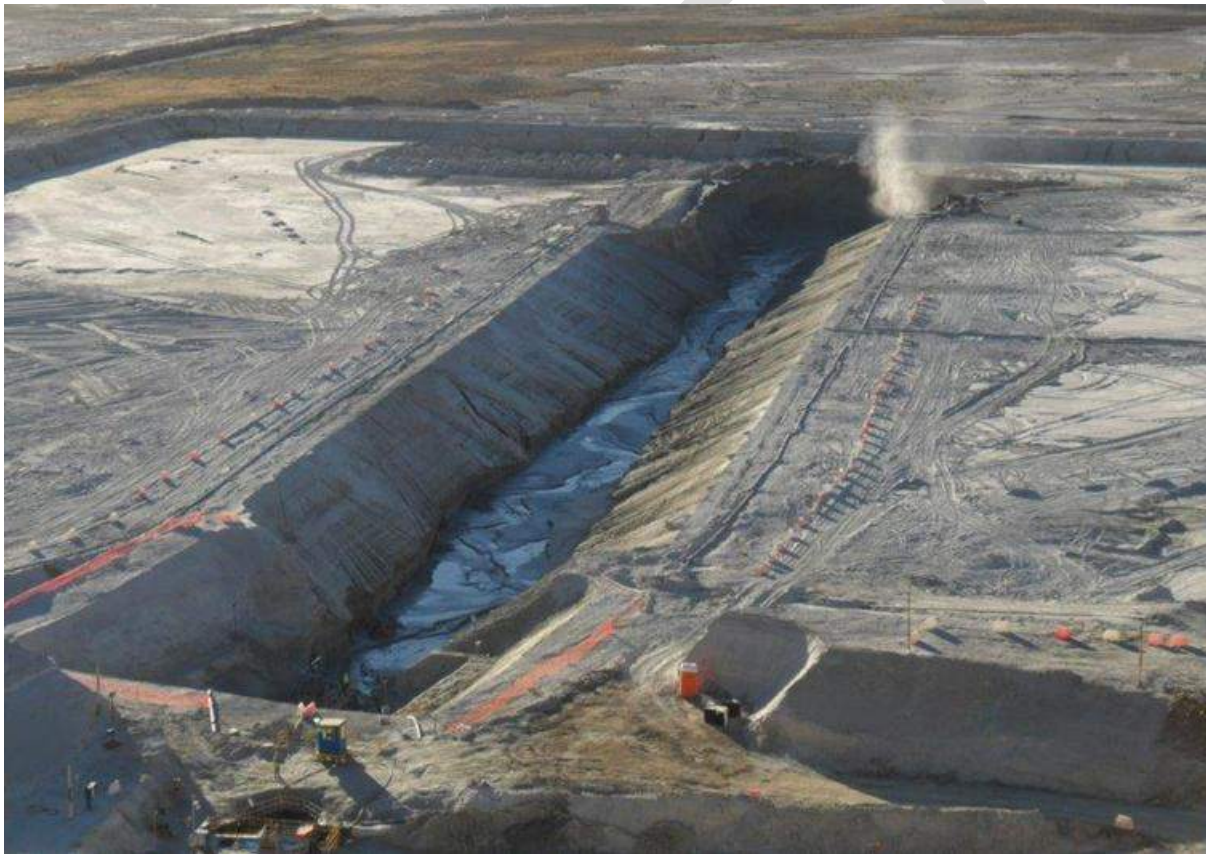
Figure 2: Typical gully being excavated via hydraulic mining methods (DRA, 2016)
