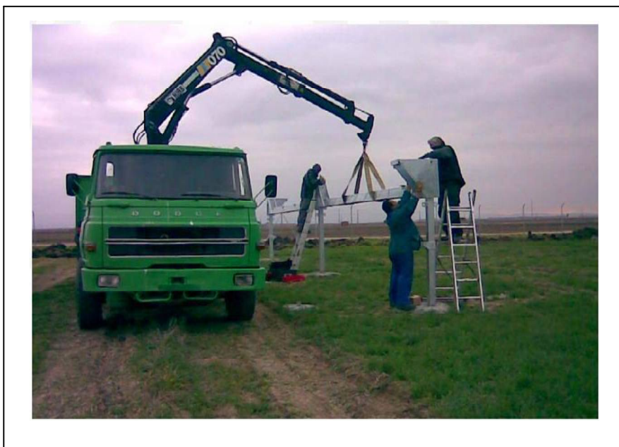
Figure 2.5 Mounting of the frame for the PV panels (Courtesy of Igeam, 2011)
