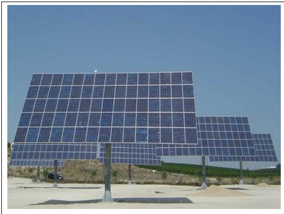
Figure 2.3: The support structures elevate the panels and allow for single axis tracking of the sun for increased efficiency (Source: energy blog)
