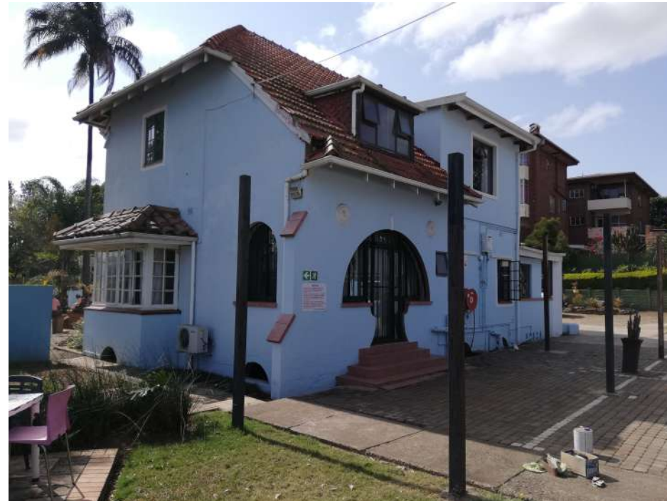
BLOCK A_ South Facing
