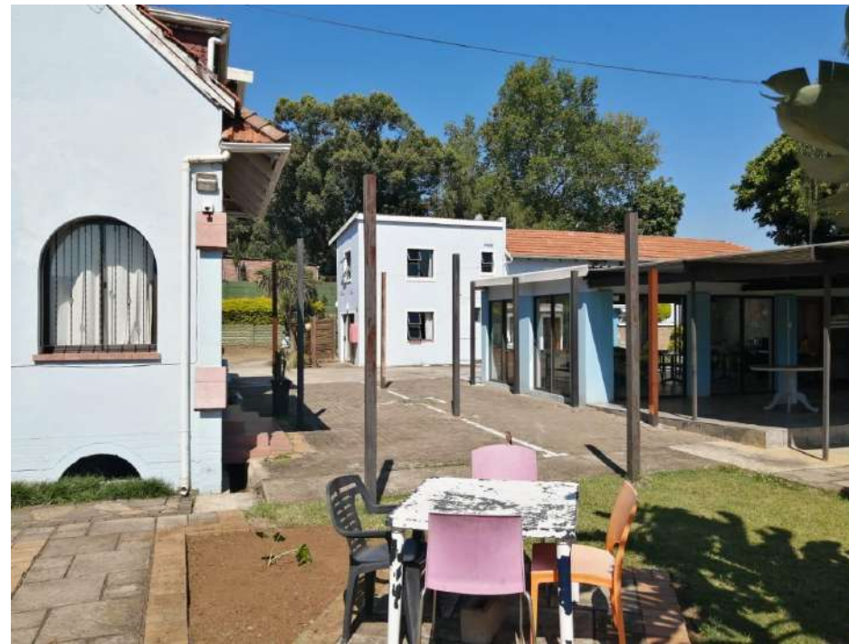
BLOCK B_ West Facing
