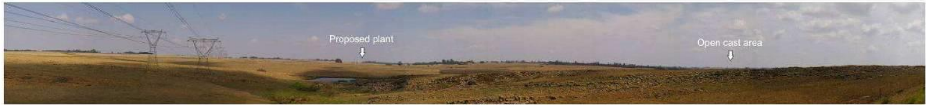
View 3: From the R33 road (Geluk-Rossow Farm) towards the proposed open cast mining area and the proposed Plant 2 site
