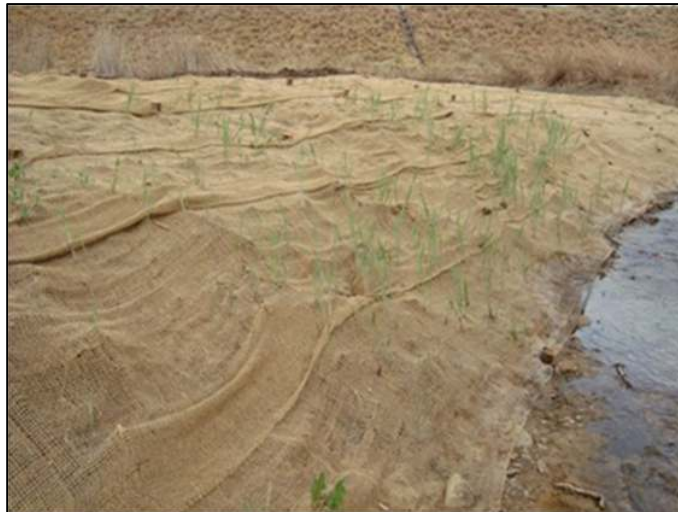
Figure 10: Geotextile used for re-seeding
