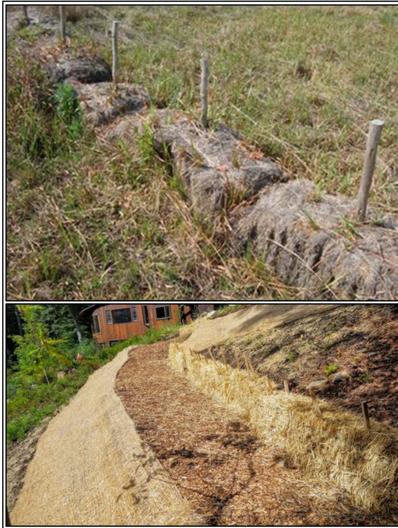
Figure 9: Pegged (staked) hay bales can be used effectively to curb soil erosion.
