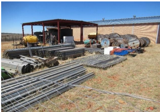
Outdoor store with WTP and water storage infrastructure
