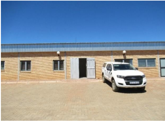
Offices and parking area
