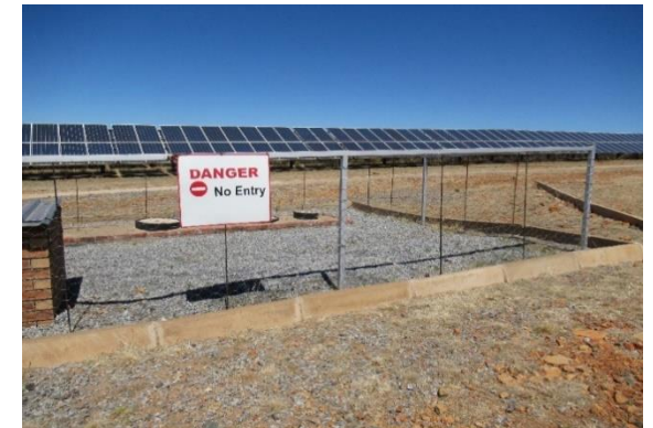
Authorised Sewage Treatment Plant (STP)
