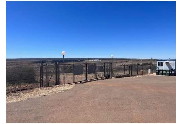
Access control to O&M buildings
