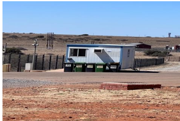
Site access control office with fencing. Waste separation evident on site
