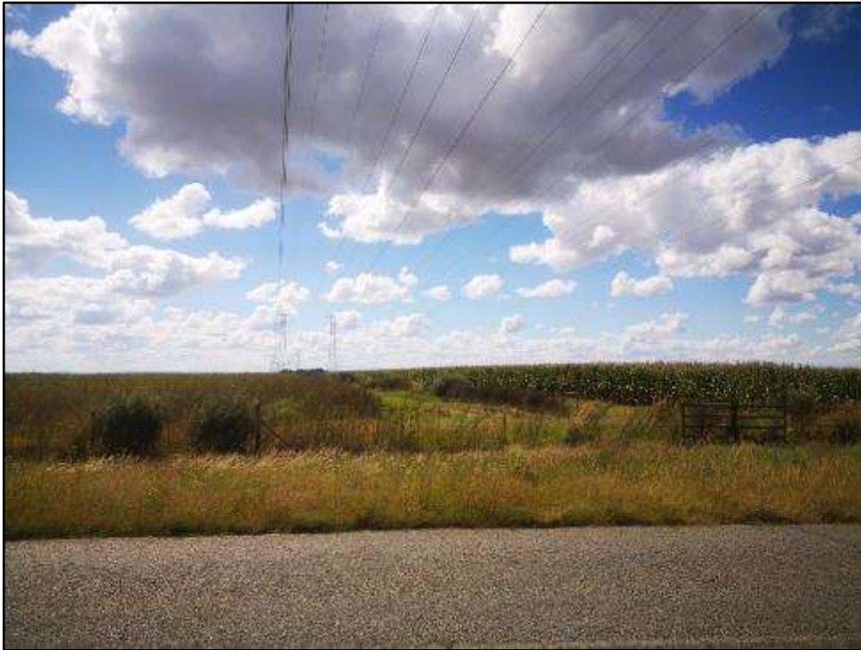
Photograph 3.10: Eskom transmission line crossing Viljoenskroon Road
