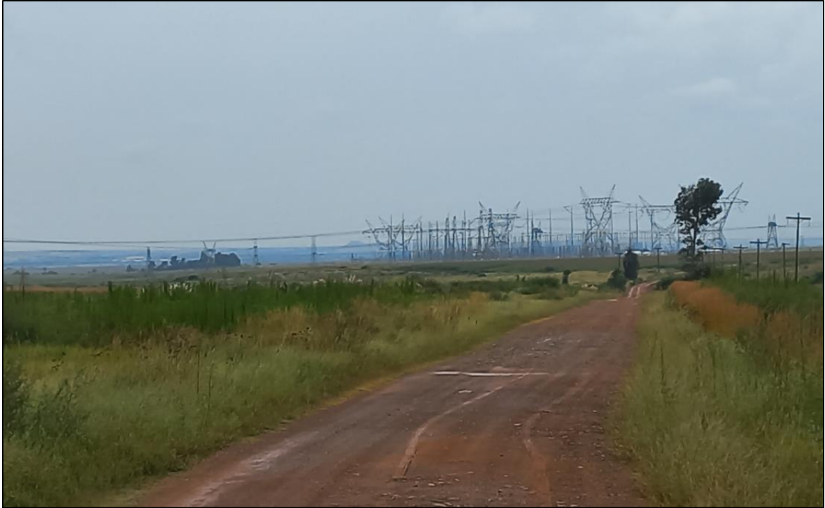
Figure 11: Photograph of the Eskom Mercury Substation.
