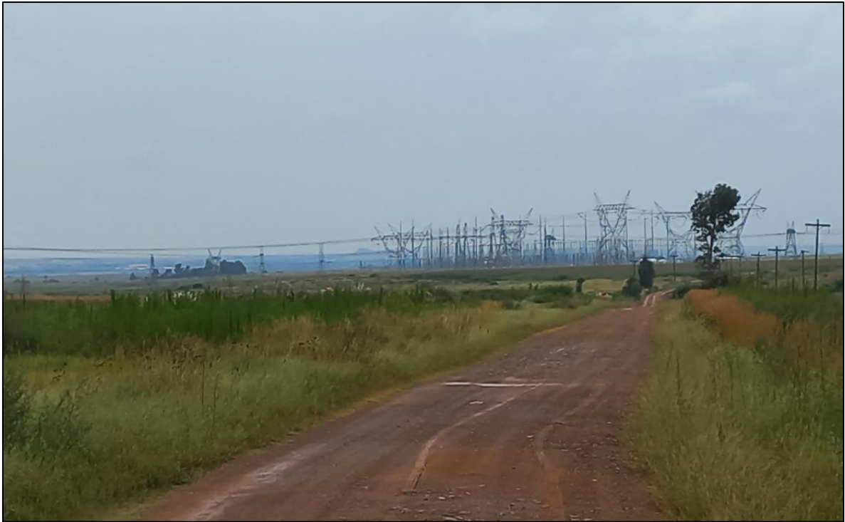
Figure 11: Photograph of the Eskom Mercury Substation.
