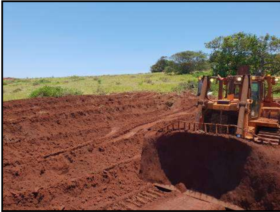
FIG.6: SITE CLEARANCE AT HT1
