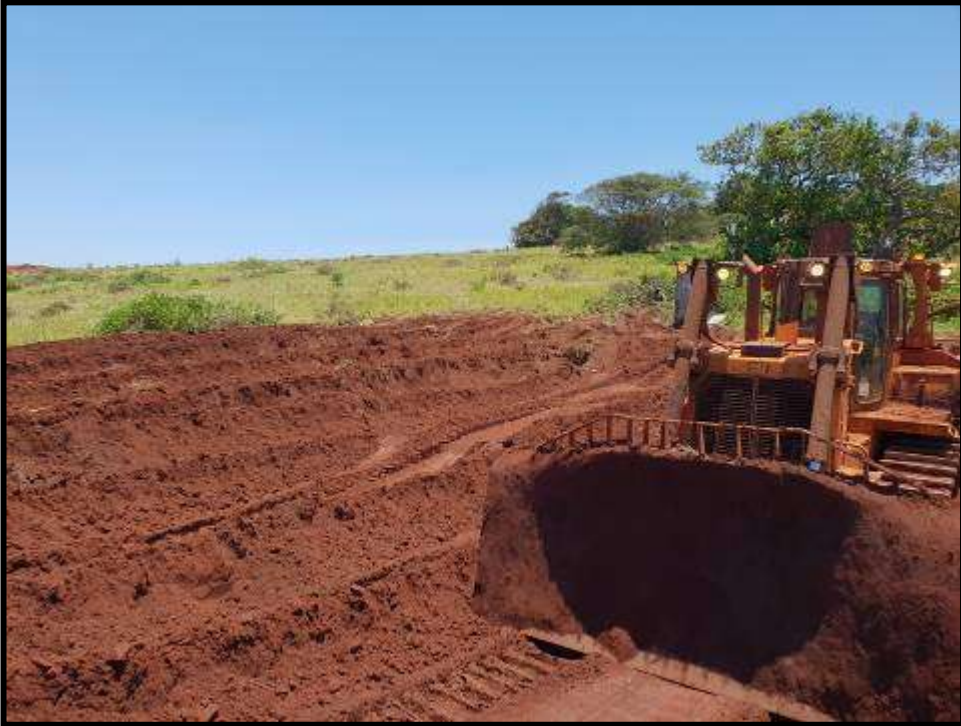
FIG.6: SITE CLEARANCE AT HT1
